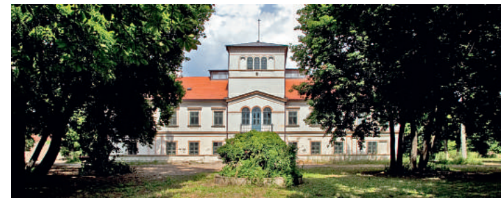
Süssenbrunn Manor in Vienna: where production of Ludwig Reiter shoes was relocated in 2011.
